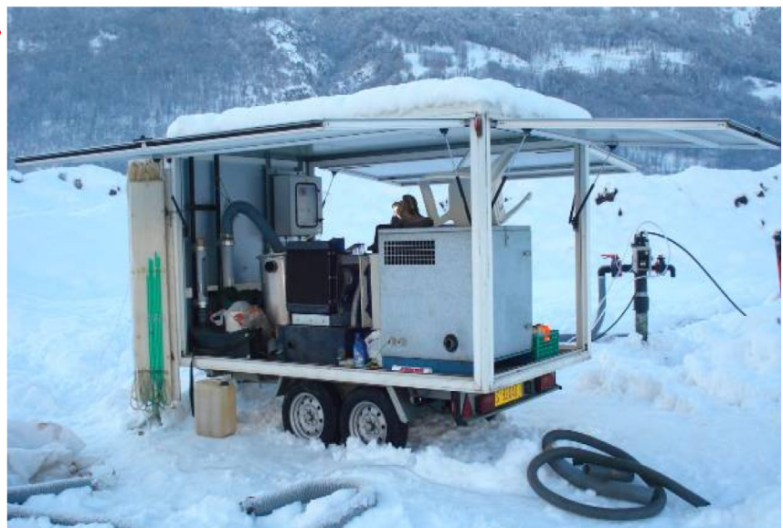
Figure 5. The air injection/gas extraction mobile unit used for the tests
