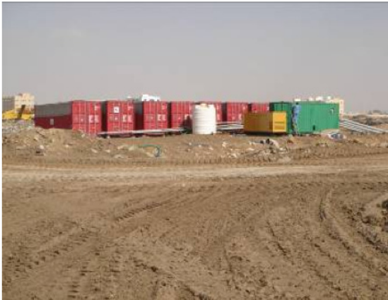
Picture 5 - Smell Well Plant
