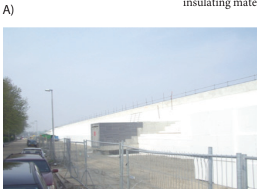
Below and right: Applications of EPS: a) light-wieght fill and frost insulation; b) bridge abutments; c) 'green' houses
