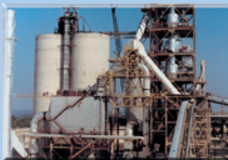
Finished cement handling and hoisting system.
