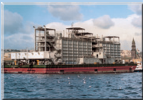
Cement handling equipment on floating pontoon.
