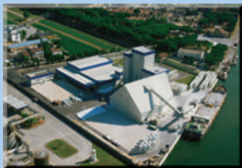
Handling equipment for premixed plaster plant.
