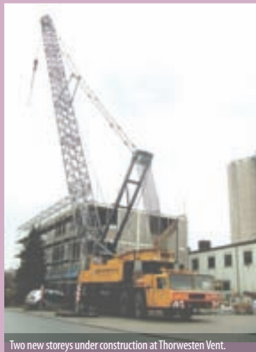
Two new storeys under construction at Thorwesten Vent.
